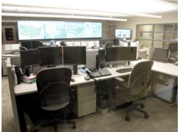
Figure 1: NOC at Batelco (Source: Wikipedia)
